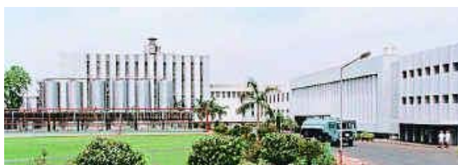
Amul plant at Anand (Gujarat)
